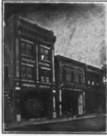
Home Office 525-27-29 N. Second St. Richmond, Va.
